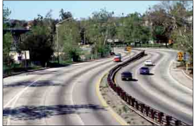
The auxiliary lane demonstration project is intended to address a need for emergency pull out areas and better transitions to on and off ramps
