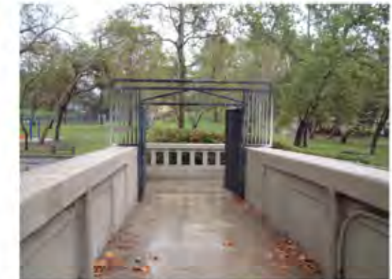
Historic Pedestrian Bridge Looking east; Hermon Run
