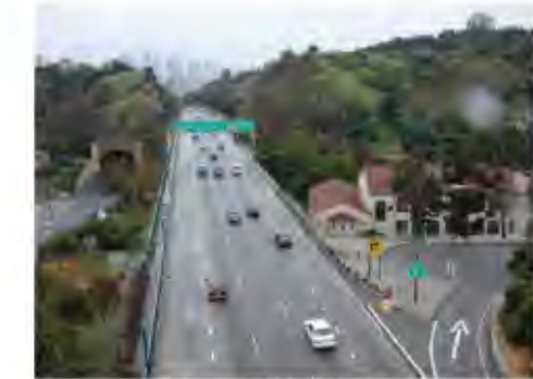
From Buena Vista Hill Bridge Looking south; Solano Valley Run
