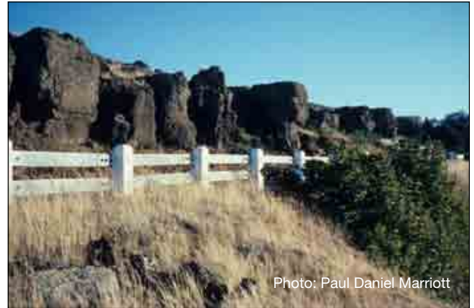
Photo: Paul Daniel Marriott Steel-backed timber barrier provided a Context Sensitive Solution for the Historic Columbia River Highway in Oregon (a National Historic Landmark highway)
