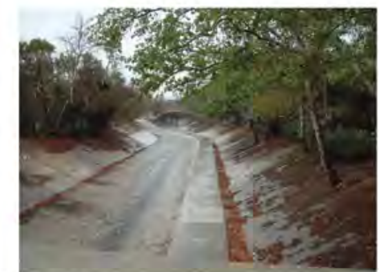
View from Pedestrian Bridge/Arroyo Seco Park Looking north; Hermon Run
