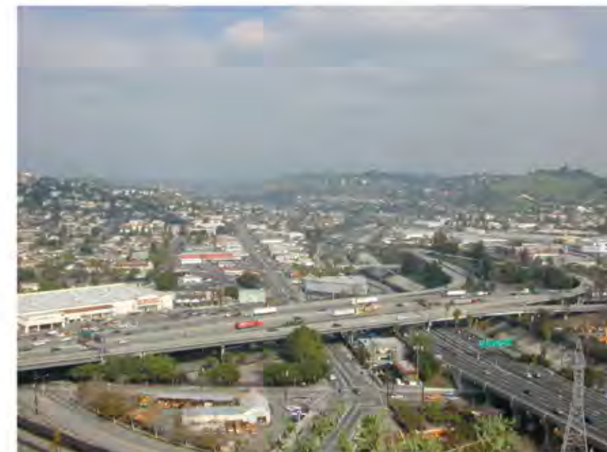
View of Arroyo Seco from Elysian Park; Portola Run, Elysian Park Reach
